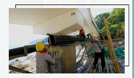
The project team swiftly mobilized for a 2-day emergency repair operation. As the concerned sewage main is located on a natural rocky shore under Mills and Chung Path with no direct vehicular or pedestrian access, the team had to build a temporary work passage and platform for carrying out emergency repair works round-the-clock.
